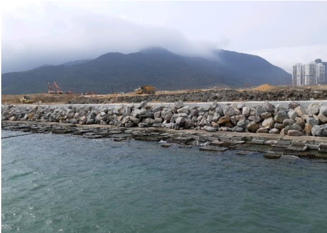
Photo 4 - Natural Rock Material/Planting for Artificial Seawall
